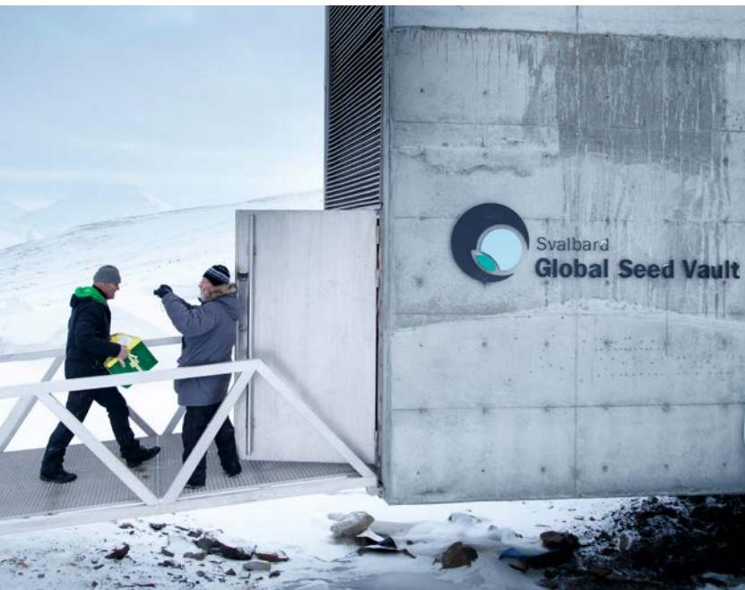
*Rectangular in shape, 54 metres long and 6.2 metres high, the Svalbard vault is carved out of a sandstone mountain, some 130 metres deep, divided into three rooms and situated at the end of a 125 metre long corridor.*
